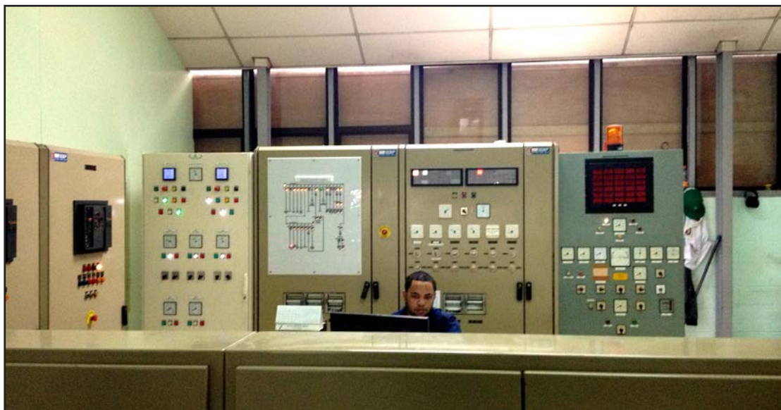
Inside the control room of the Avatiu Power Station
